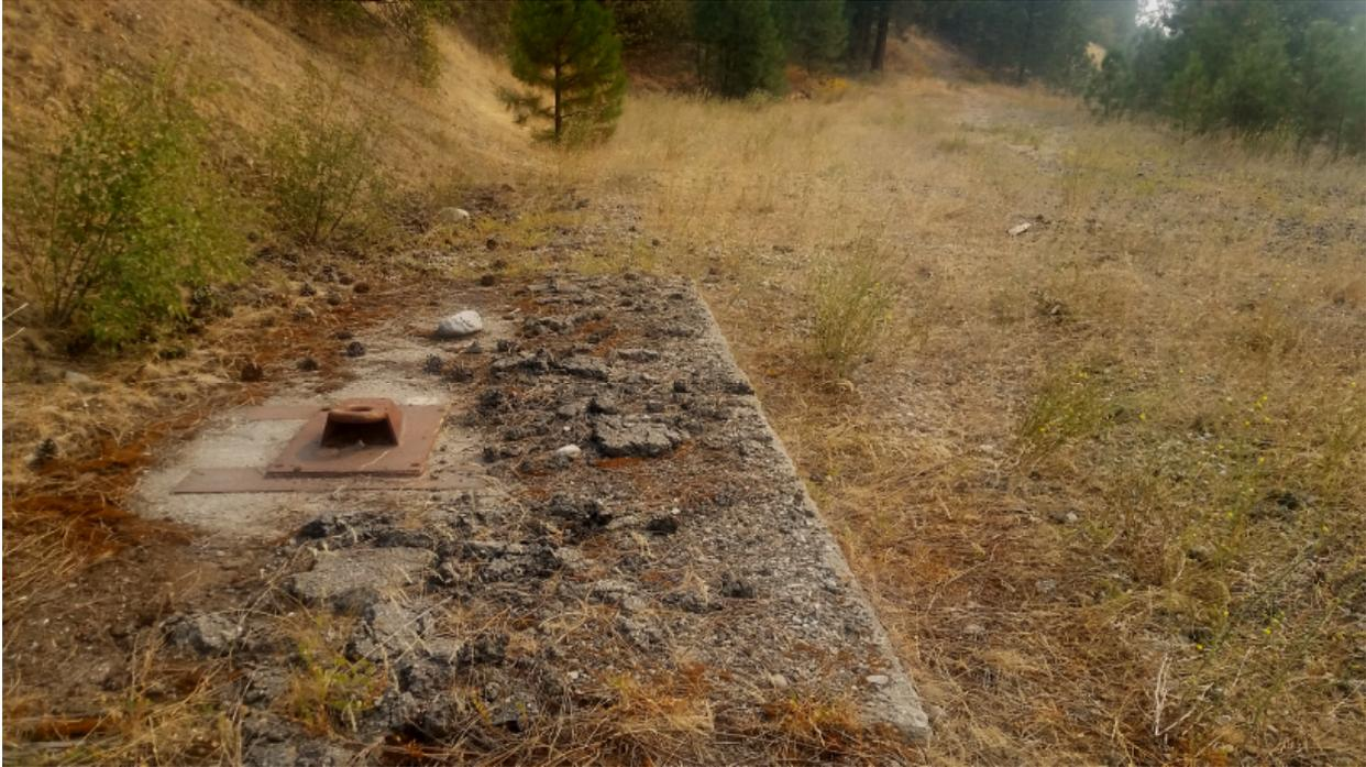
**Photo 17:** Looking east at a former winch anchor point along railroad ROW or a spur line. The device was used to move railcars.
