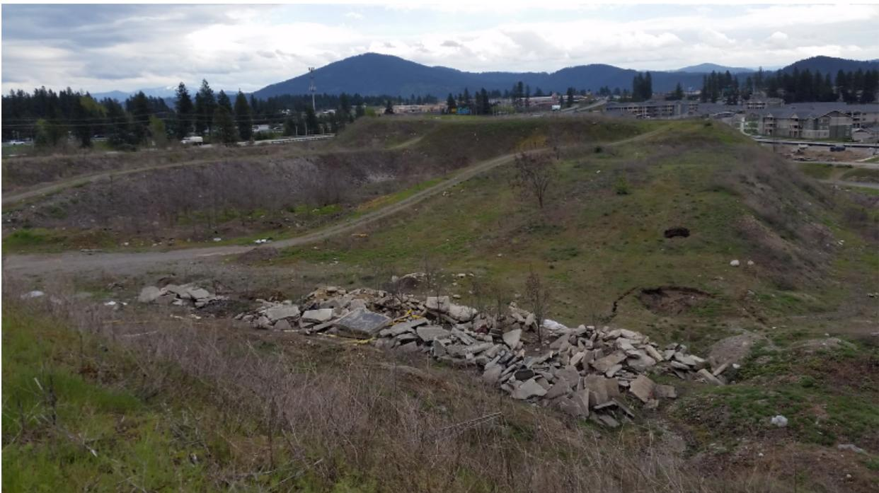
**Photo 8:** Panning right and looking easterly at the wood waste stockpile that also includes concrete debris. Subsidence is notable within the stockpile, which rises as much as 60 feet above surrounding landscape.
