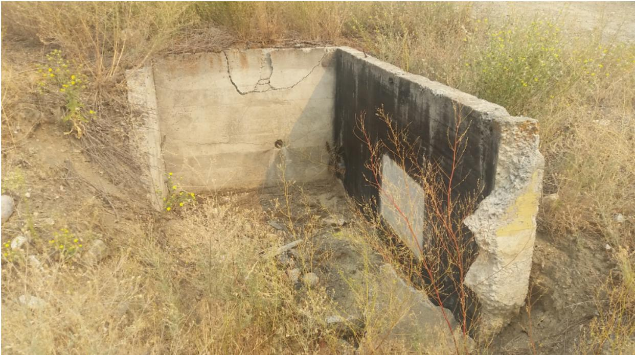
**Photo 14:** Looking at a former septic tank once located near the northern end of the sawmill building. Clay tile pipe was observed leading to this feature.
