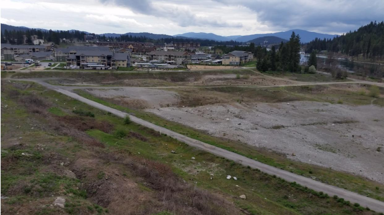
**Photo 1:** Looking southeast across the former lower log storage area on site (see **Figure 3**) and the former ROW of the NPRR. The area was scraped of top soil and debris, which was stockpiled on the northeast portion of the site. The Riverstone residential development and the North Idaho Centennial Trail are in the background.
